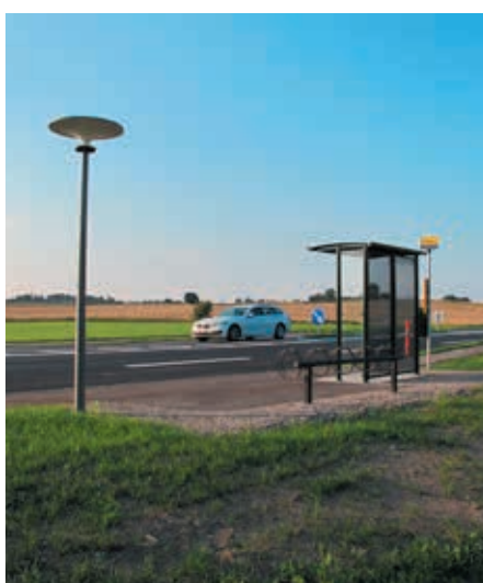
Denmark – Asima® Sun, Standalone, In cooperation with Gribskov Municipality
